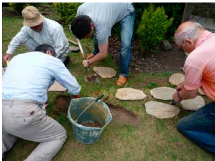
During the works
